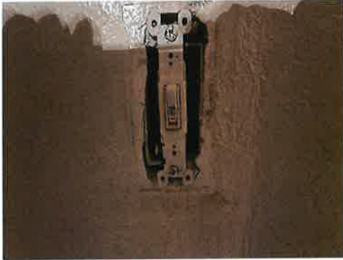
1218-1 Plaster Typical Interior Walls/Ceilings
