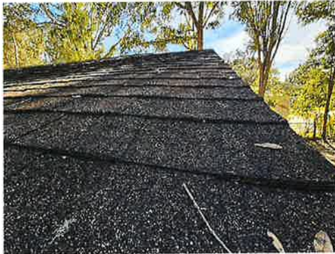
1218-3 Asphalt Shingle/Tar Typical Exterior Roof
