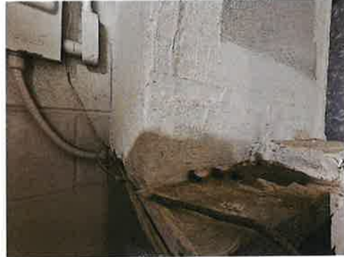
1218-2 Duct Mastic Typical Interior HVAC
